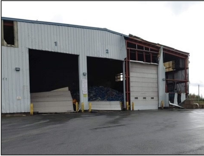
Materials Recovery Facility in Kempton
