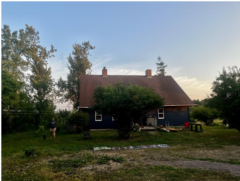
McCurdy Creek House, rear view
